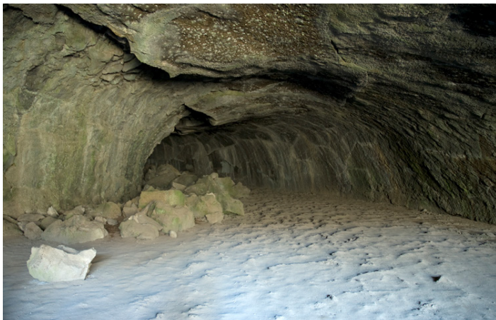
Fallen Rocks Blocking Entrance of Mine Tunnel
